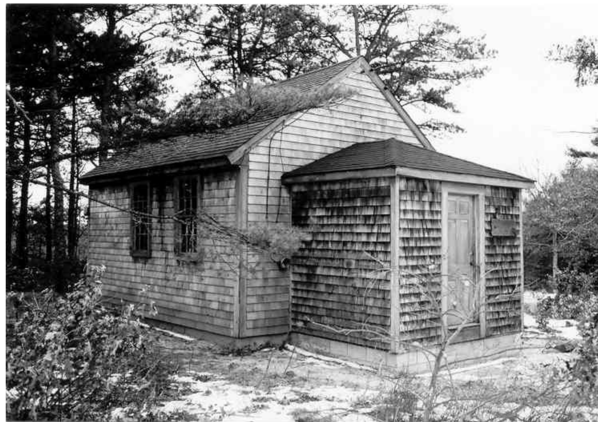
South Mashpee One Room School House (1831 - 1901)
